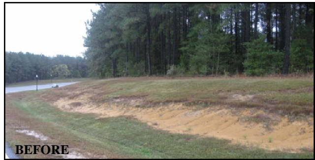
Excessive mowing on this steep slope led to scalping and rutting by the landscape crew. The goal of this planting was to remove the mower from the maintenance equation and break-up the length of the slope.
