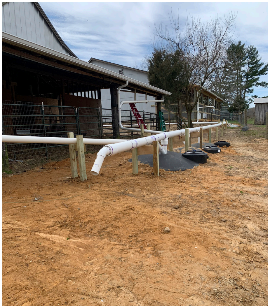
Right: A portion of the finished rainwater harvesting system. The building in the previous images is shown in the background, and a second building included in the system is in the foreground. The cisterns storing all of the captured water are buried between the two buildings. Pumps are used to pump water out of the cisterns when needed.
