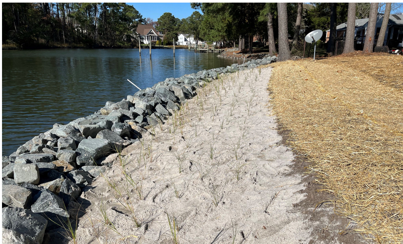
This image shows the same shoreline as above after a living shoreline has been installed. During installation, a sill was built out of large stone, sand was added to build up the new marsh area, and marsh grass plugs were planted to help stabilize the sand. Over time, these marsh grasses will fill in the length of the shoreline and provide water quality and habitat benefits.
