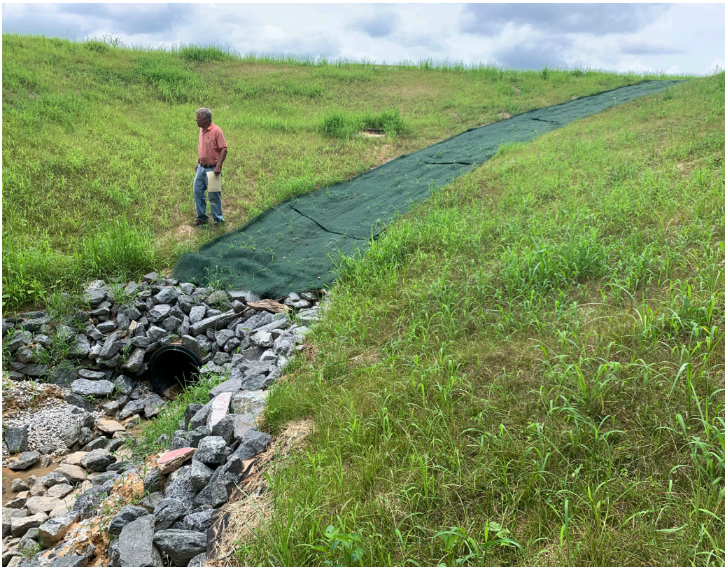
The landowner surveys the completed project after slopes have been stabilized with EC-3 matting and seeded.
