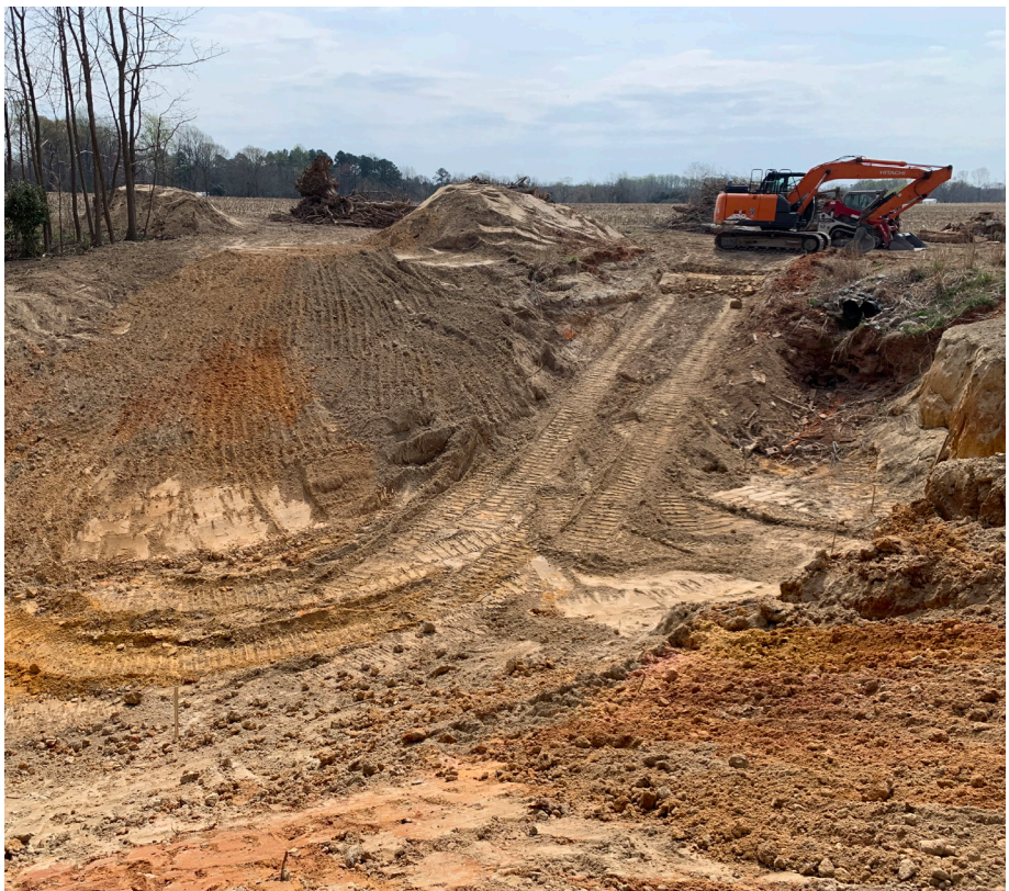
Site preparation and earth moving/smoothing. Slope grades must be prepared before laying pipe or stone.
