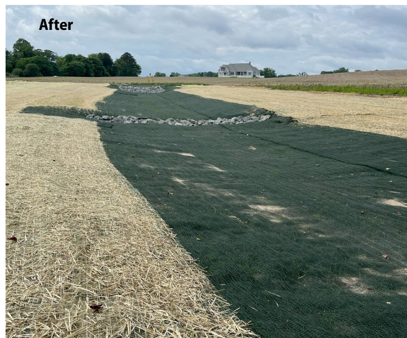
Figure 3. The significant erosion (left) prior to the installation of the lined chute (right).
